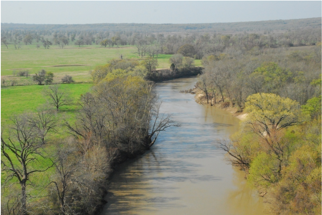
Figure 2-5. Trinity River Crossing (Facing South)
